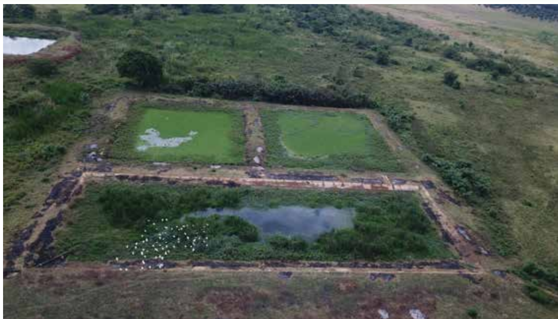
Plate 18: EMC Waste stabilisation ponds (One facultative pond and two parallel maturation ponds) (Photo taken in August 2023)
